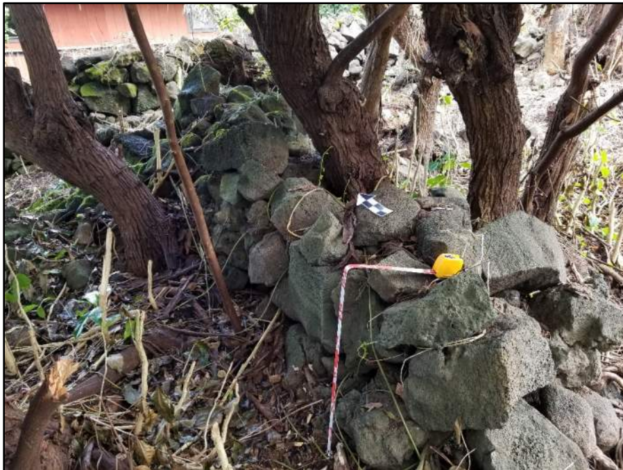
Figure 101. Photo of SIHP # -31124 terrace wall; view to northeast
