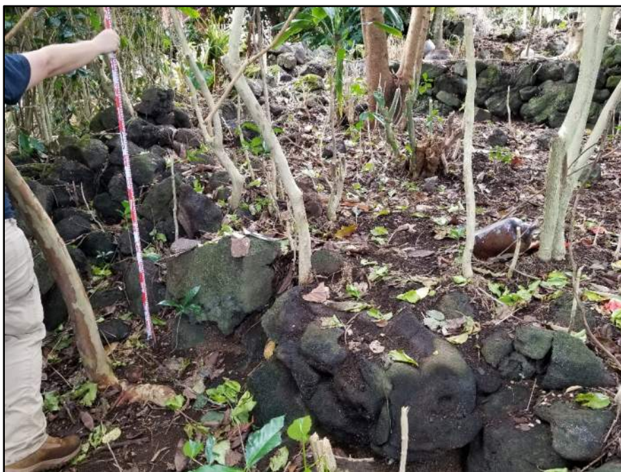
Figure 115. Photo showing the SIHP # -31124 Feature I terrace wall and terrace behind, at the interface with Feature A mauka-makai wall; view to northeast
