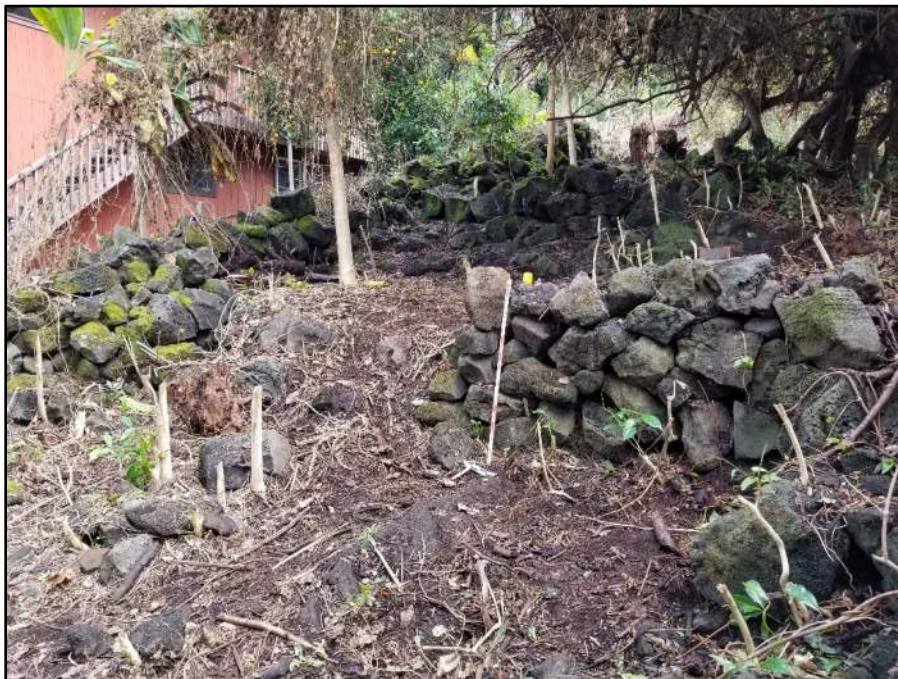
Figure 105. Photo of the northern portion of the SIHP # -31124 Feature D terrace wall and terrace behind; view to northeast
