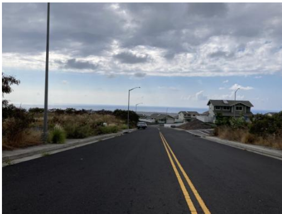
Photo facing west showing road with several completed houses in La'i 'Ōpua
