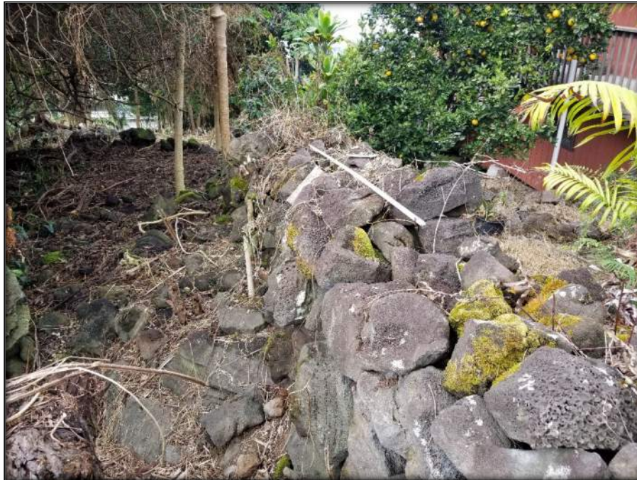
Figure 98. Photo showing a portion of SIHP # -31124 Feature A mauka-makai wall; view to west
