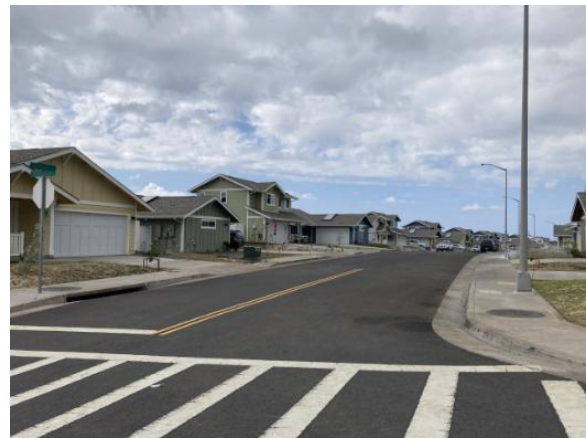
Photo facing north-west showing fully developed residences
