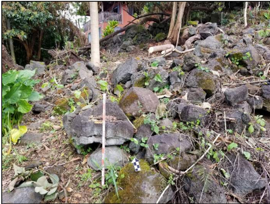
Figure 112. Photo showing the impacted southern portion of the SIHP # -31124 Feature G terrace wall; view to north
