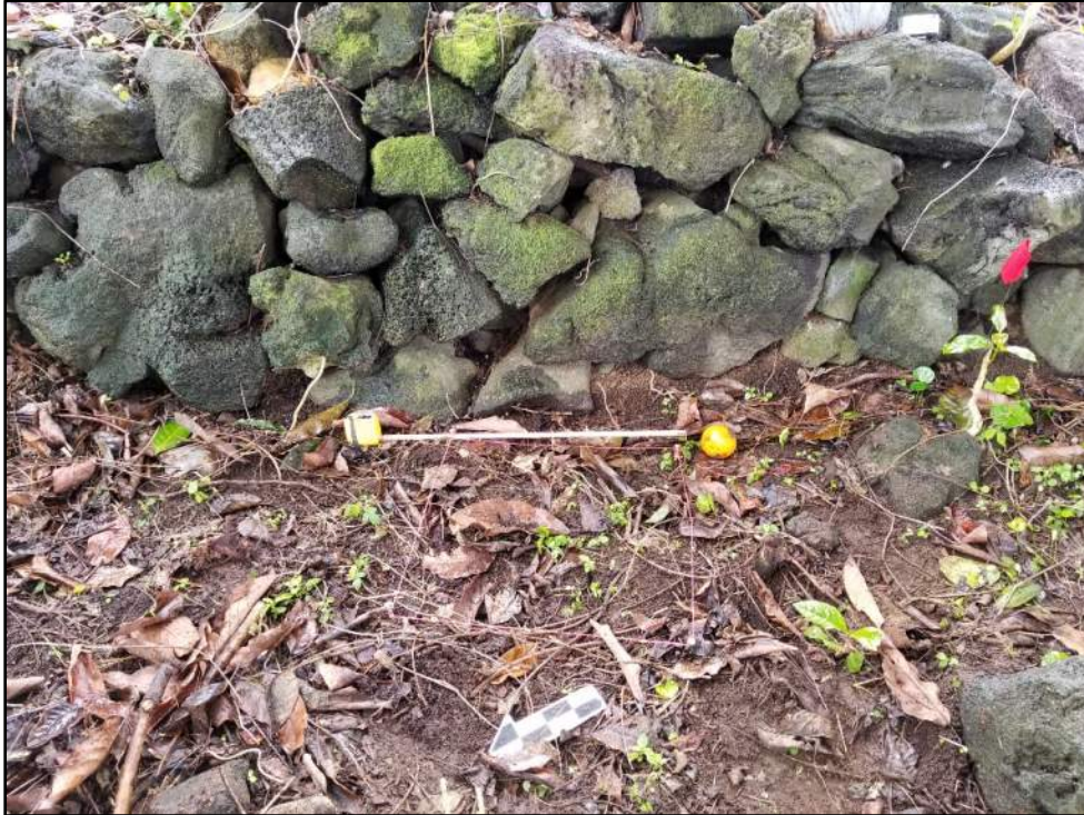
Figure 35. Photo of TU-3 marked out with pink string prior to excavation; view to southeast
