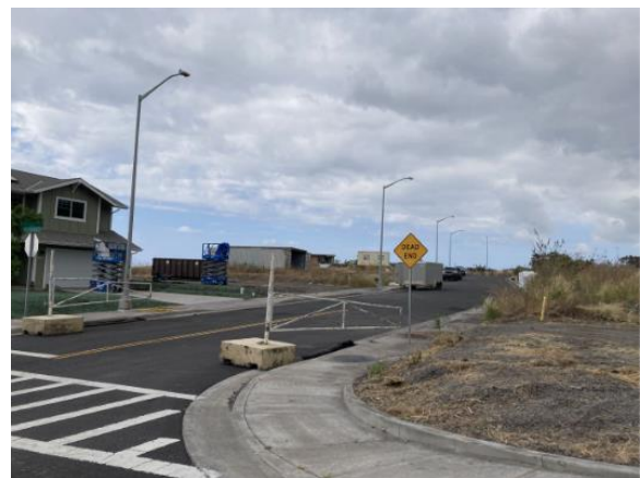
Photo facing north-west showing a portion of community under construction
