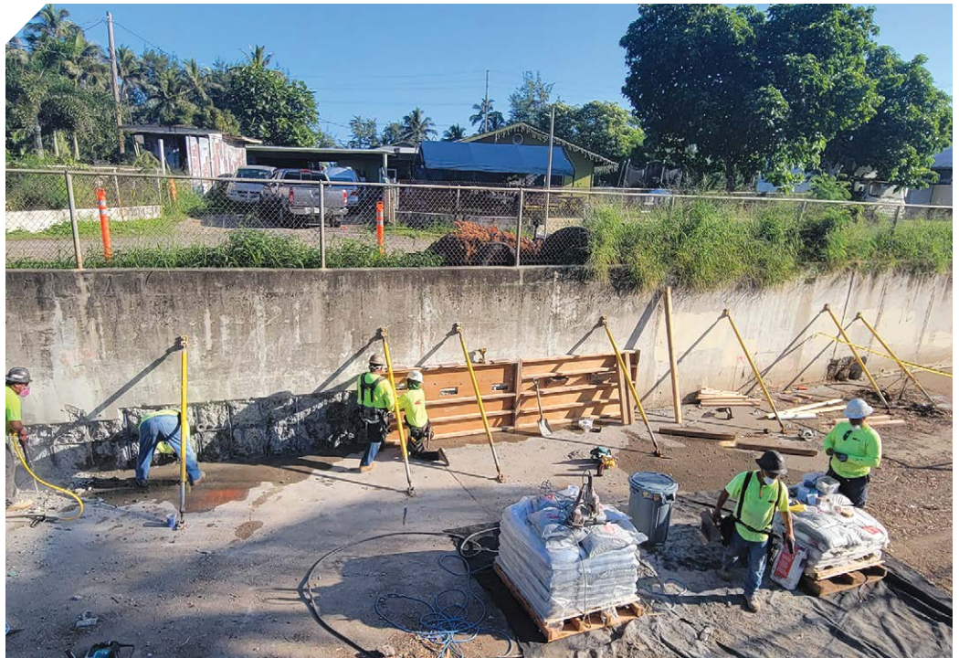
▶ Waimānalo Flood Drainage Channel Improvements - O'ahu
