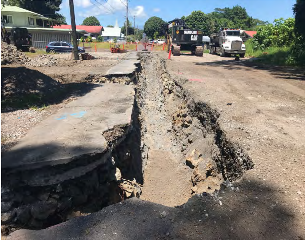
Trenching for rerouting DWS waterline affecting several sewer laterals
