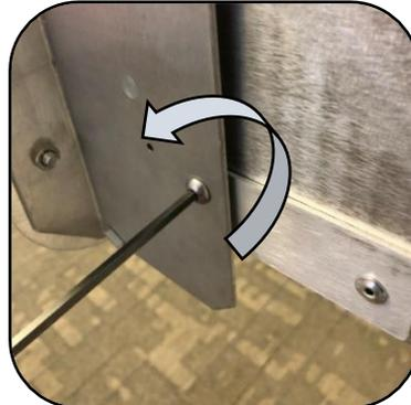
Remove the two fasteners
