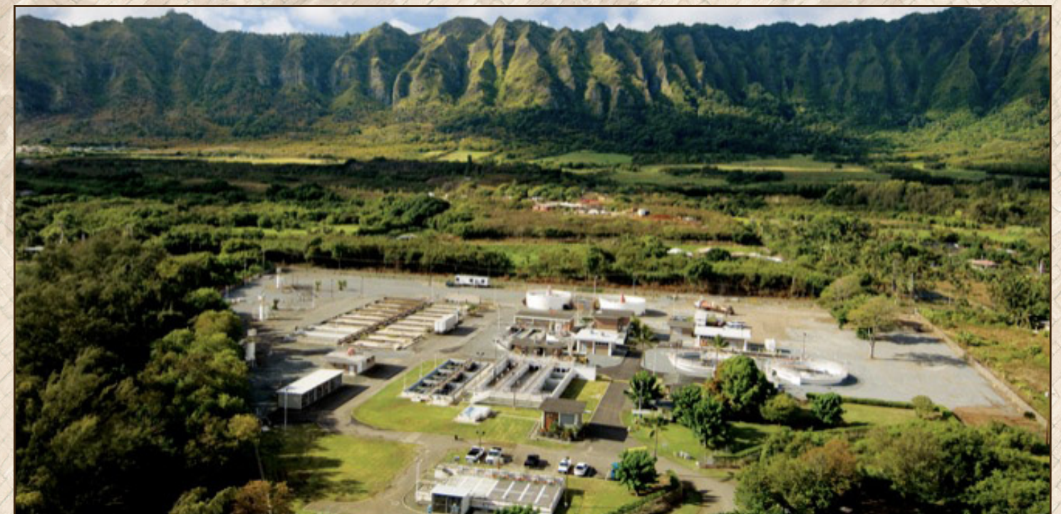
Waimānalo Wastewater Treatment Plant
