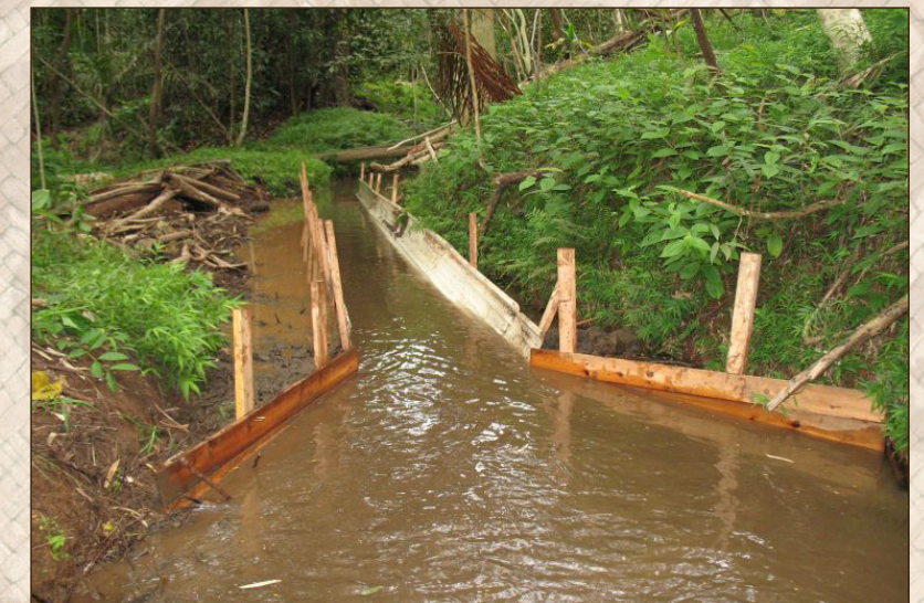
Temporary Repairs at Maunawili Ditch
