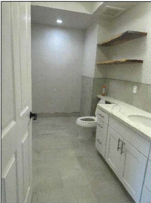
Newly renovated bath (tub not installed)
