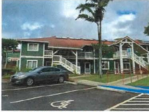
TYPICAL EXTERIOR VIEW OF APARTMENTS
