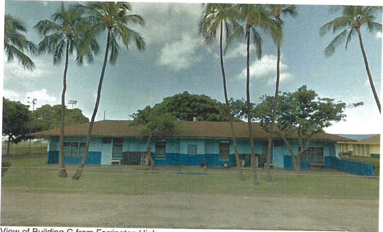
View of Building G from Farrington Highway.
