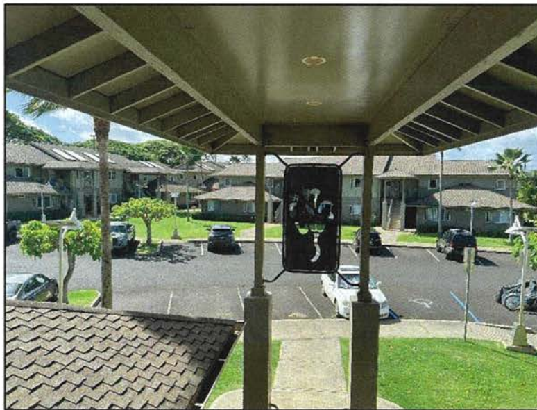
View from second floor stair landing.
