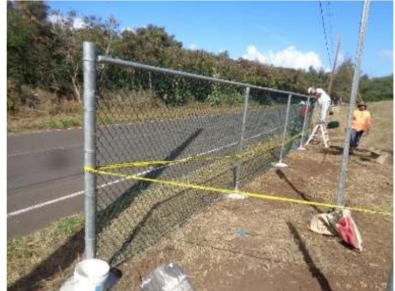
Contractor installing a 6 foot chain-link fence along Halewaiu Road
