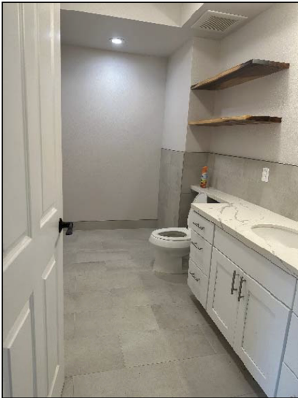
Newly renovated bath (tub not installed)
