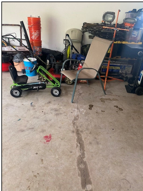
Foundation crack in garage; tenant reports rock walls along homesite have also sustained damage as a result of settlement
