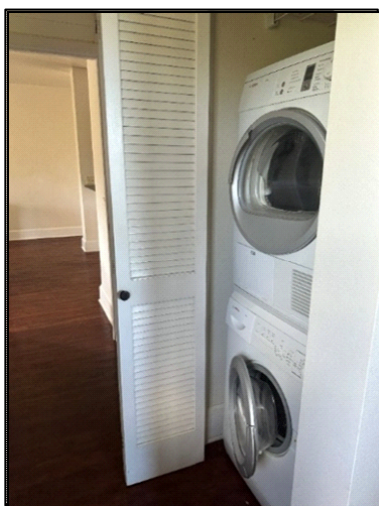
In unit stack laundry
