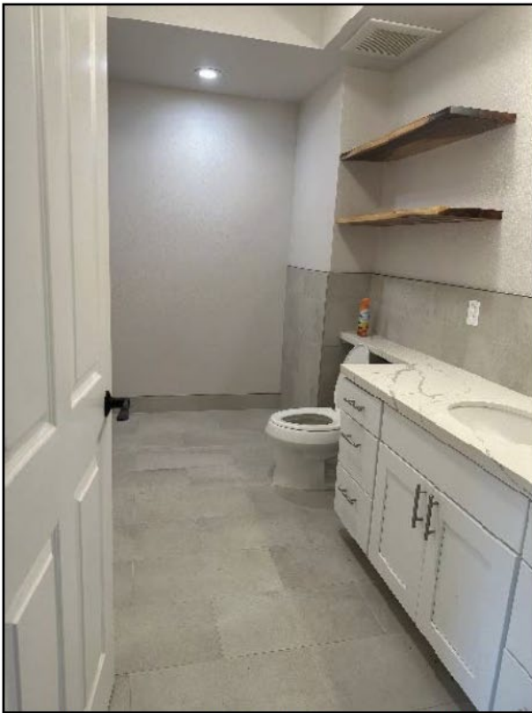
Newly renovated bath (tub not installed)
