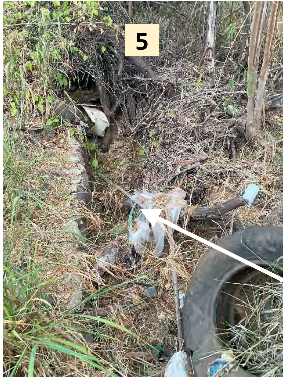
Drainage ditch full of rubbish parallel to road that is not able to serve its drainage function which could cause flooding on the road, the church and the school.
