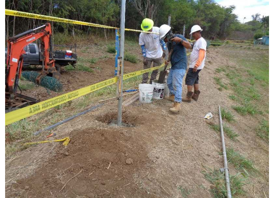
Contractor mixing concrete for fence post footing
