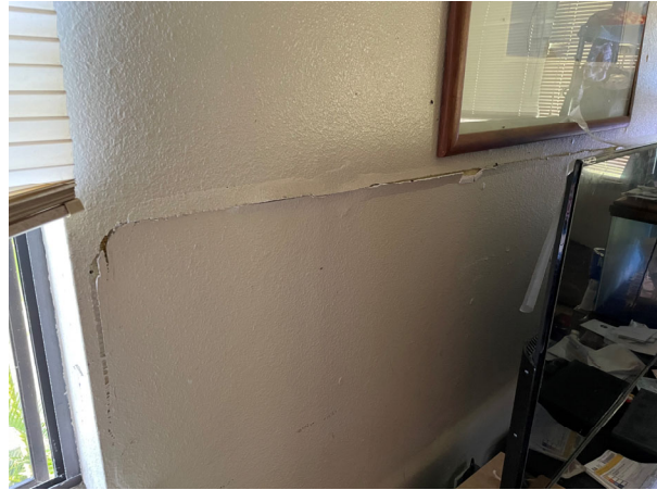
Cracks in the interior walls
