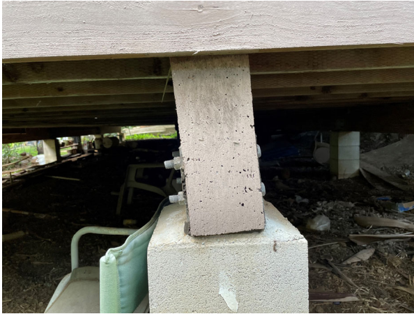
Shifting structural post
