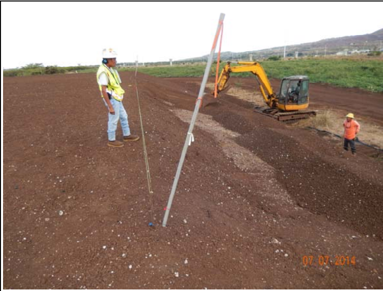
Photograph 28: Placement of top soil in preparation for hydroseeding.
