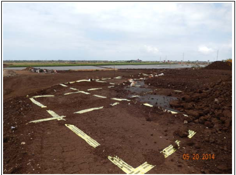
Photograph 25: View of metallic tape placed above contaminated soil (thin layer of soil between orange construction fencing and metallic tape).
