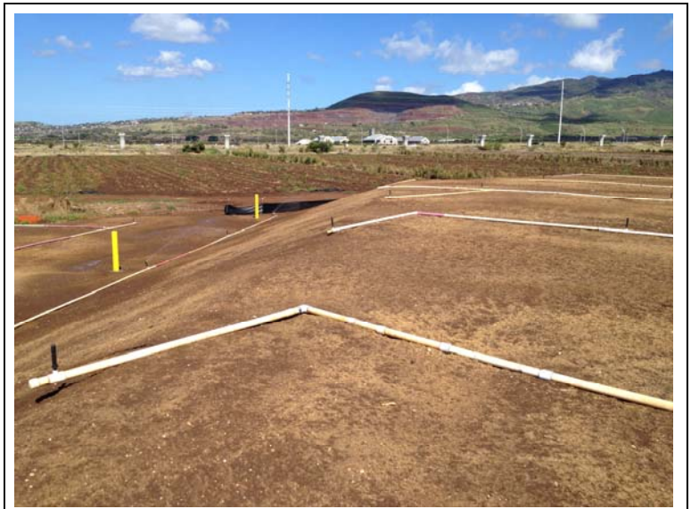
Photograph 35: View of irrigation system installed after hydroseeding.
