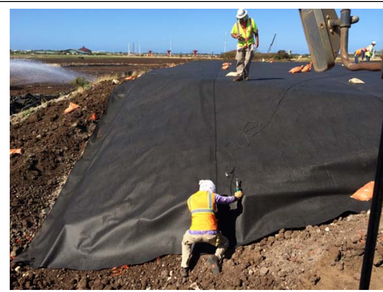
Photograph 15: Welding and securing geomembrane liner.
