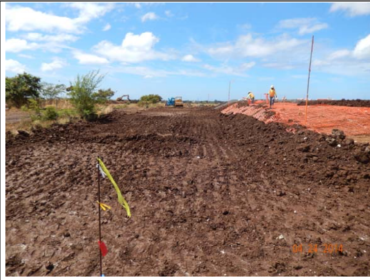
Photograph 22: Backfilling and compacting excavation area adjacent to PML fill area.
