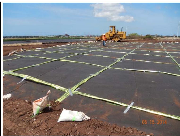
Photograph 24: Placement of metallic tape using 10-foot grid spacing.
