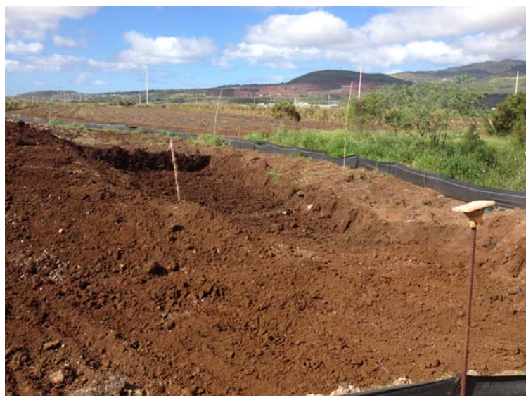
Photograph 10: View of excavation area north of PML boundary.
