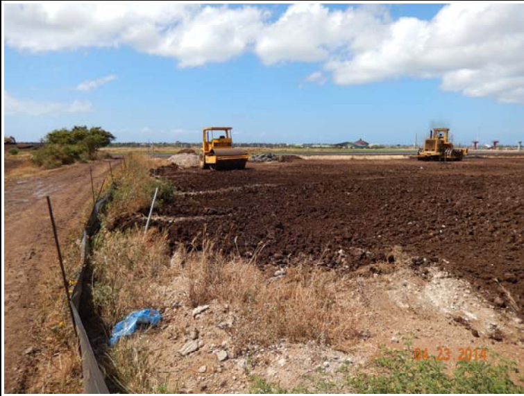
Photograph 19: Backfilling excavation area outside of PML boundary.
