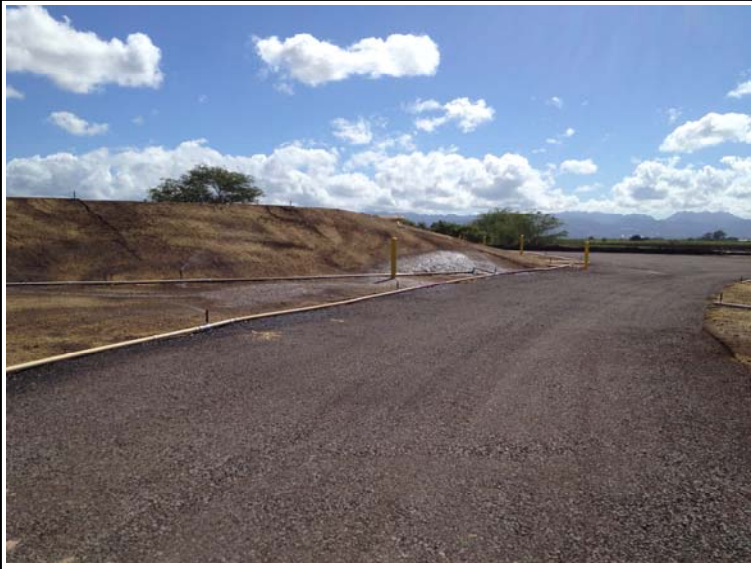
Photograph 34: View of site after completion of backfilling and hydroseeding.
