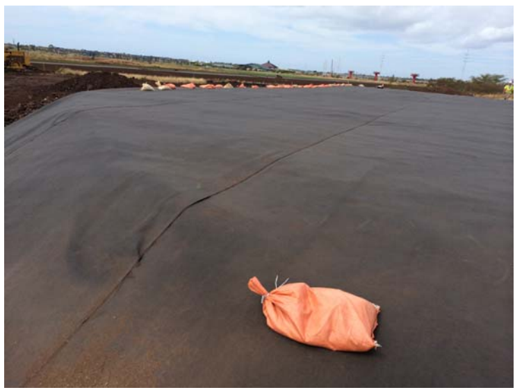
Photograph 16: View of geomembrane liner, welded and anchored in placed.
