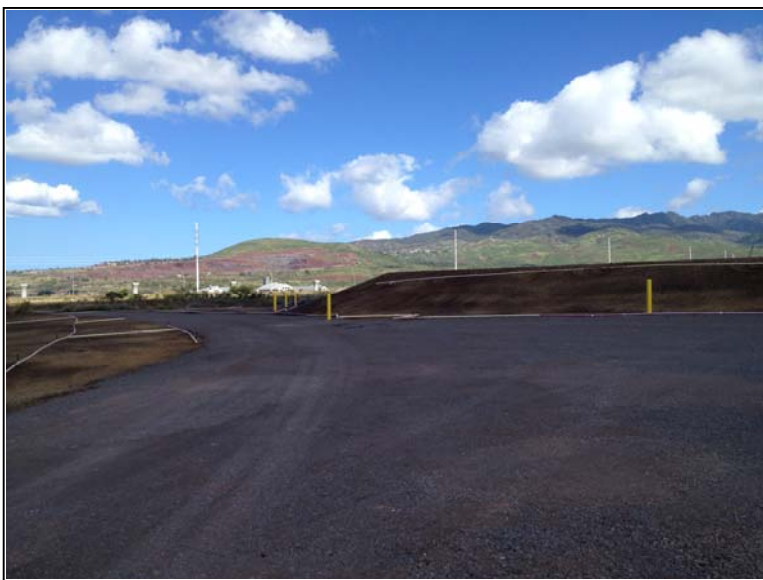
Photograph 33: View along haul road following backfilling and hydroseeding.
