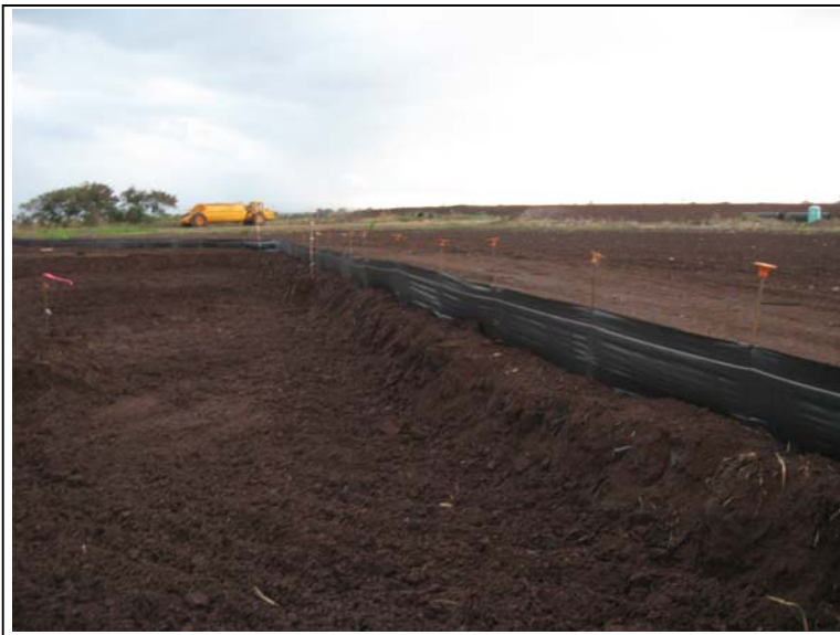
Photograph 3: Start of soil excavation outside of PML boundary.
