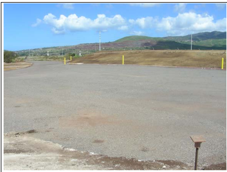
Photograph 33: View of granular fill used to re-establish haul road.
