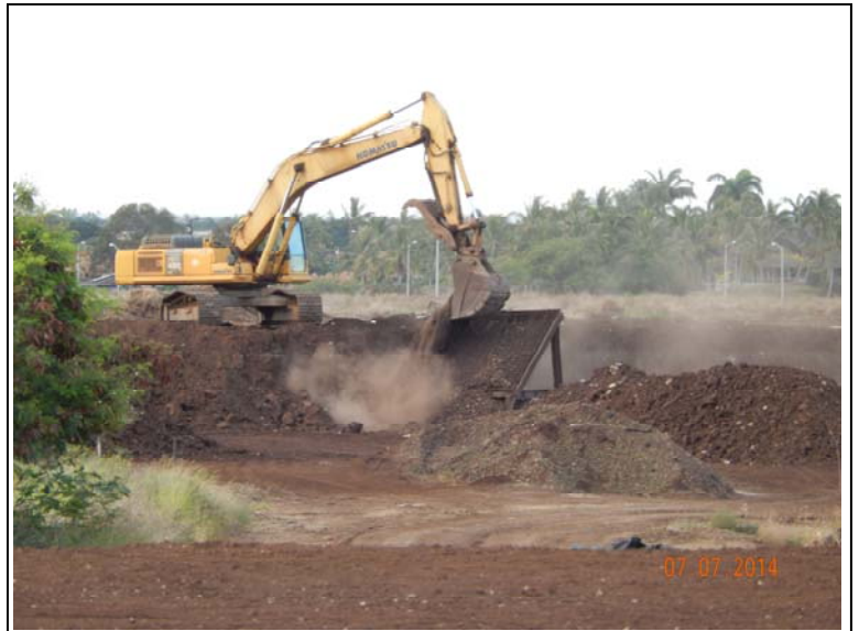
Photograph 29: Screening soil at borrow site to meet specifications for top soil.
