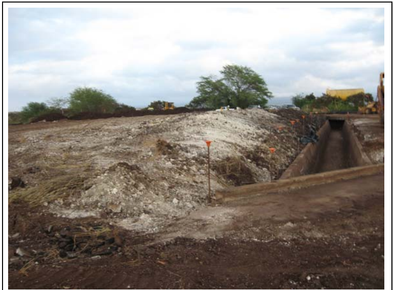
Photograph 5: Soil removed from section of concrete-lined irrigation ditch adjacent to PML site.
