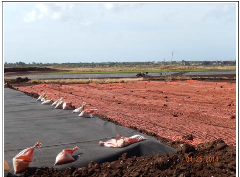
Photograph 23: View of geomembrane liner and visual indicator barrier.
