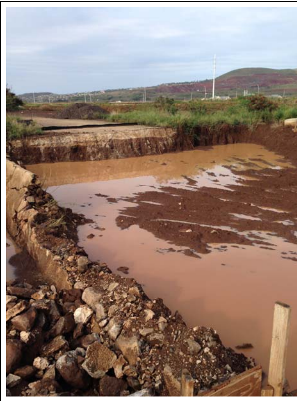
Photograph 9: View of excavation area outside of PML boundary.
