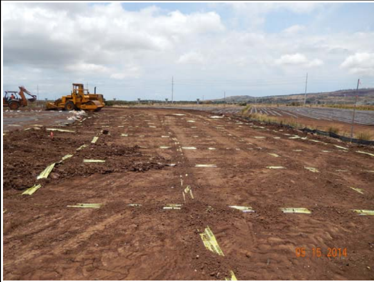
Photograph 25: View of metallic tape placed above contaminated soil (thin layer of soil between orange construction fencing and metallic tape).
