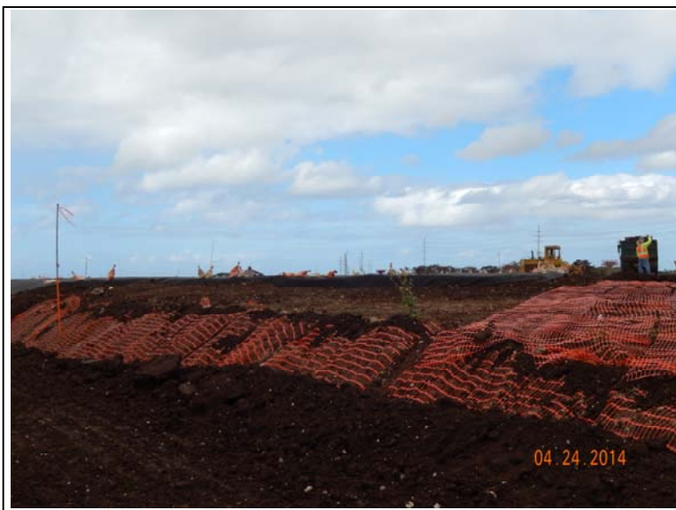
Photograph 21: Orange construction fence used as visual indicator barrier.
