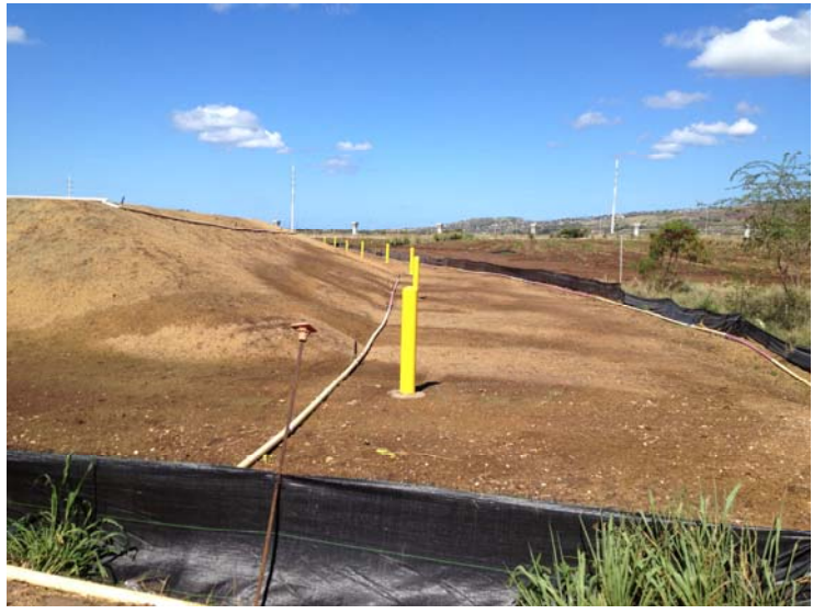
Photograph 31: View of concrete-filled pipe bollards. Hydroseeding complete, irrigation system installed.
