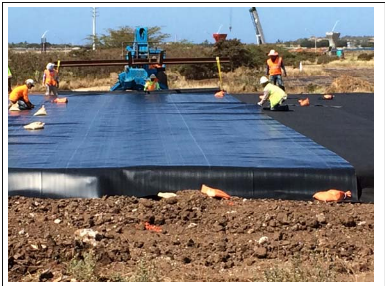
Photograph 14: Placement of geomembrane liner.
