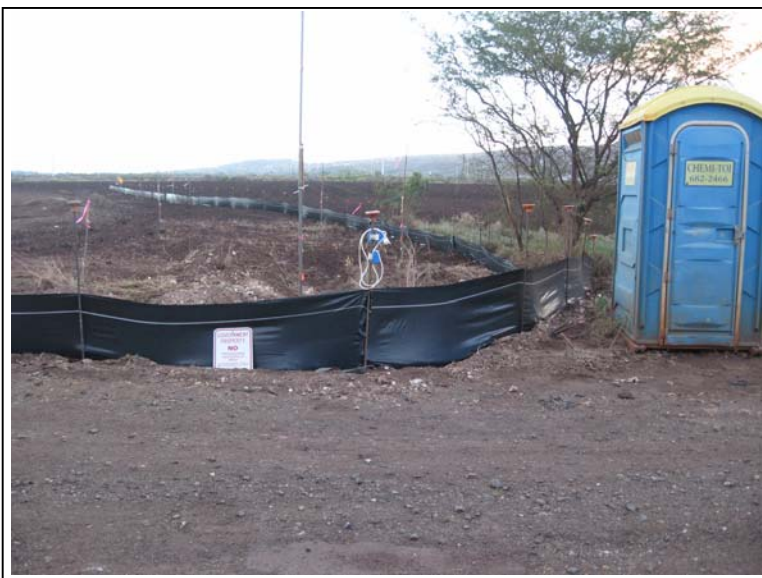
Photograph 6: View of typical pump and media used for air monitoring at project boundaries.
