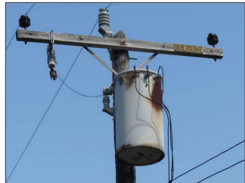
FIGURE 1. AN AGING ELECTRICAL TRANSFORMER ON MCKINLEY STREET AT THE PARK
