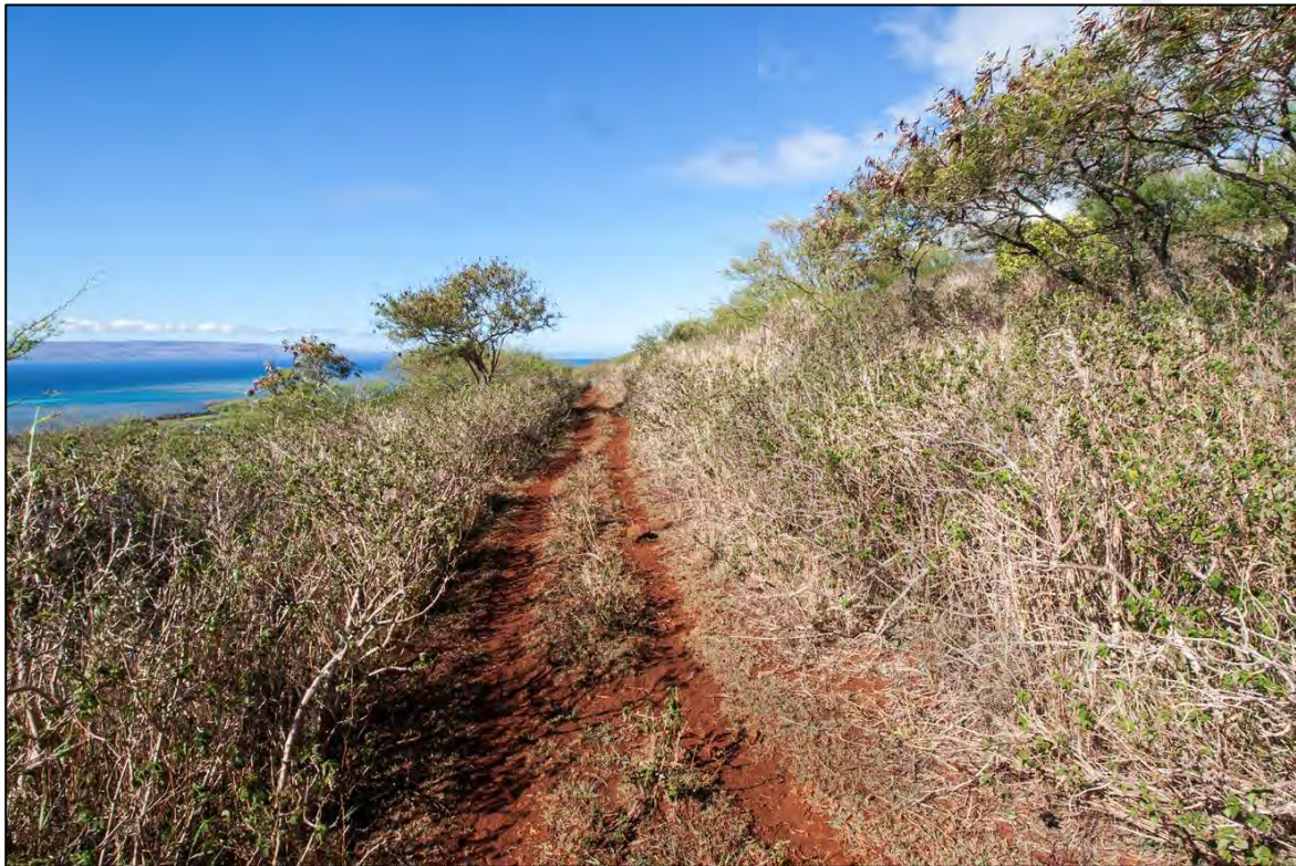
Figure 15. Portion of same road as in previous figure, but here constructed along the contour. Road is still traversable by vehicles and is a minor contributor to slope erosion and reef degradation.
