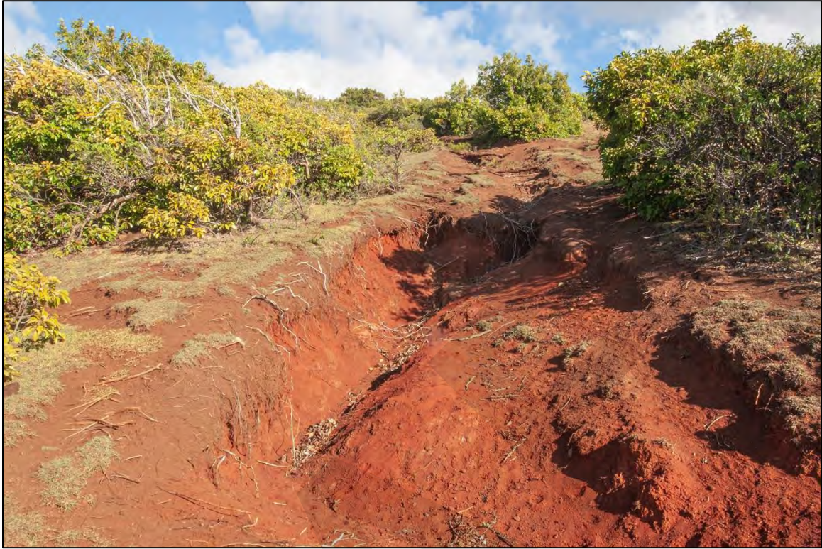
Figure 14. Portion of a former road constructed across the contours and now a site of extensive erosion. Road is no longer useful for vehicles.
