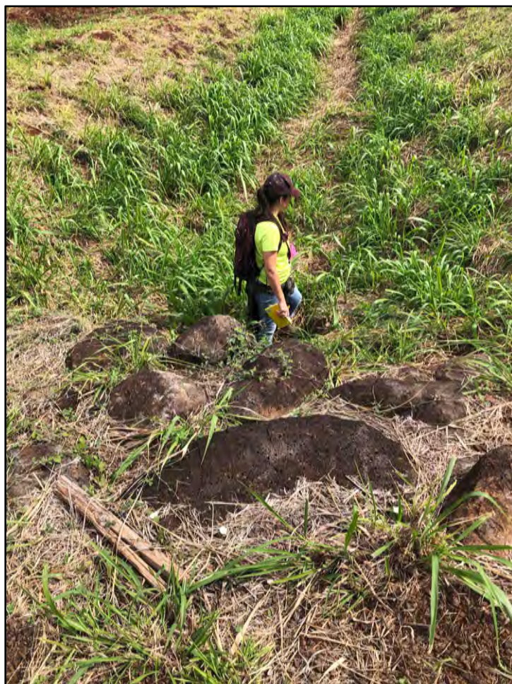
Figure 29. Atop the culvert looking down and makai.
