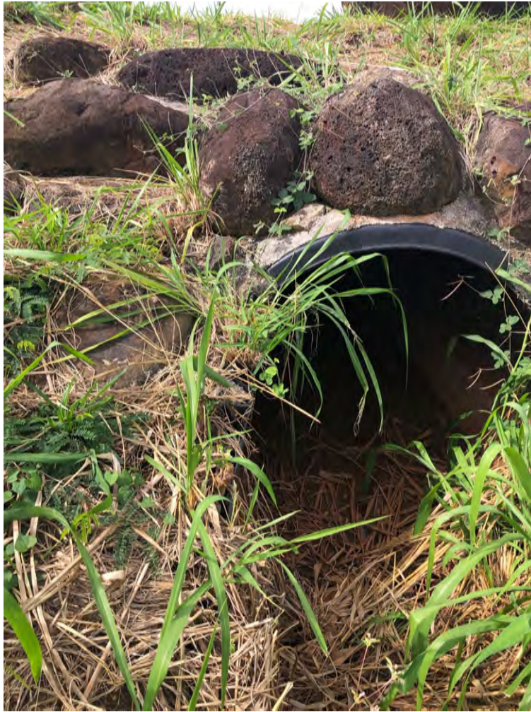
Figure 28. Showing the culvert
