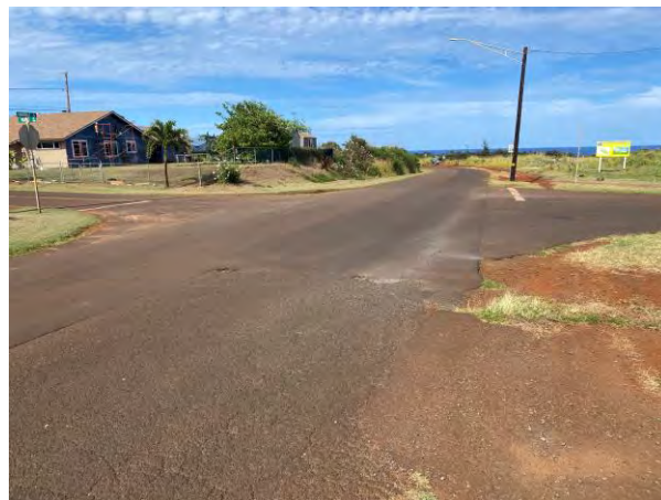
Figure 3: Existing Kukuihale Road/Pilipoli Road Intersection
