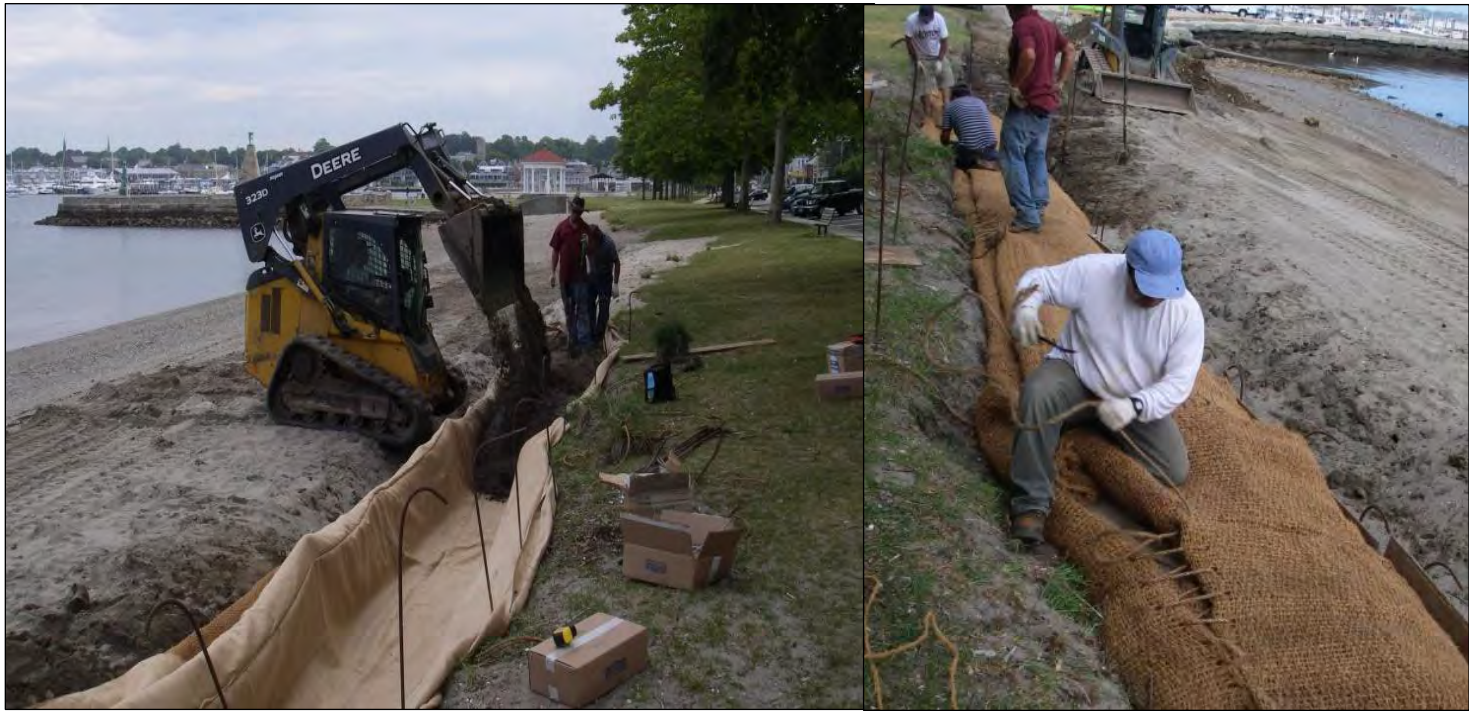
Photos: Examples of a sand-filled coir ‘burrito’ at King’s Park, Newport, RI Photos courtesy of Janet Freedman (TNC, 2017).
