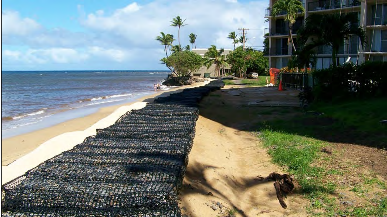
Photo: Tensar geotextile mattress filled with hard, angular rocks to capture sand particles.
