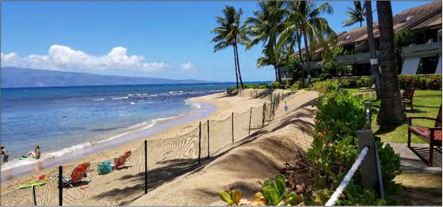
Photo: Sandy berm with a sand-filled coir burrito before planting at Kahana Bay, Maui, HI.
