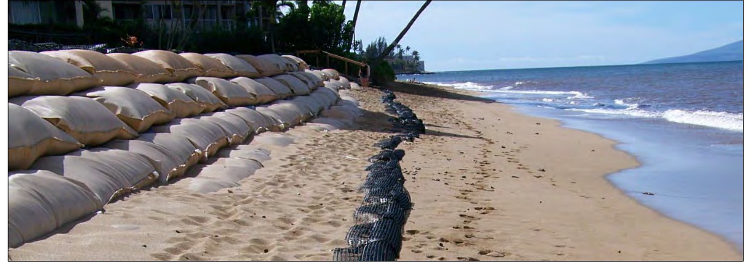
Photo: A sand-filled Elco brand geotextile bag revetment atop Tensor mattresses, West Maui.
