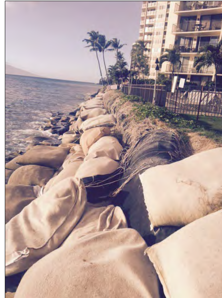
Photos: Geotextile bags may shift due to storm surge and typically require maintenance over time as these before and after photos illustrate, West Maui.
