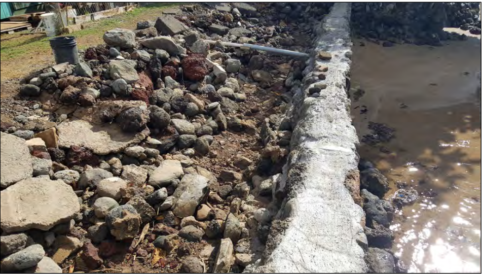
Photo: This wall’s effectiveness could be improved with more weep holes distributed behind the wall and more porous aggregate as fill.
