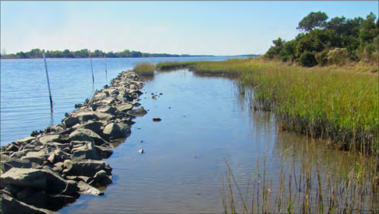
Photo: Breakwater sill and marsh vegetation at Morris Landing, Holly Ridge, NC. Photo: Carter Smith . Source: https://ncseagrant.ncsu.edu/currents/2018/11/living-shorelines-can-enhance-saltmarsh-resilience-to-hurricanes/
