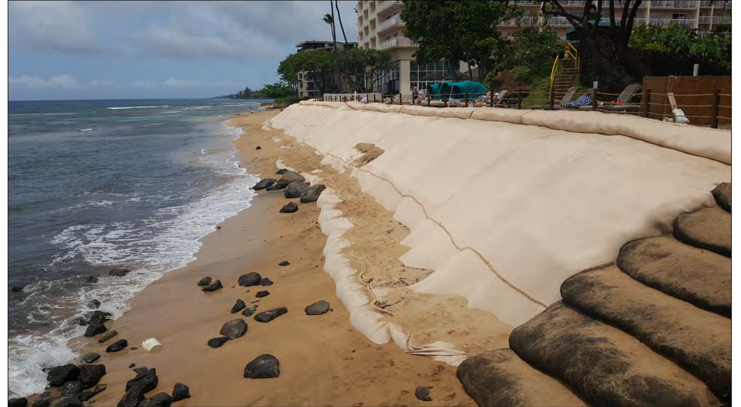
Photo: A geotextile erosion skirt covering an eroded embankment at the Kā’anapali Beach Club, West Maui, 2018.
