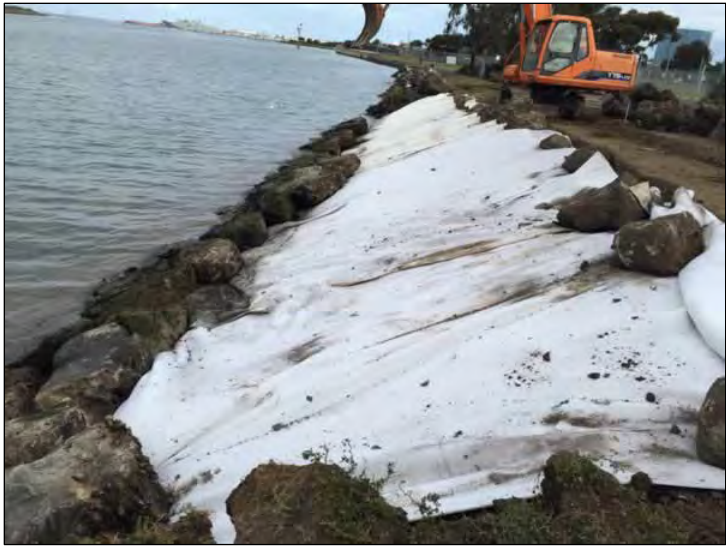
Photos: A properly designed revetment has interlocking stones underlain with geofabric.
