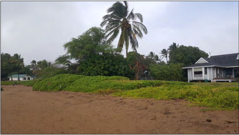
Photo: A vegetated sand berm protects a house from waves and flooding.
