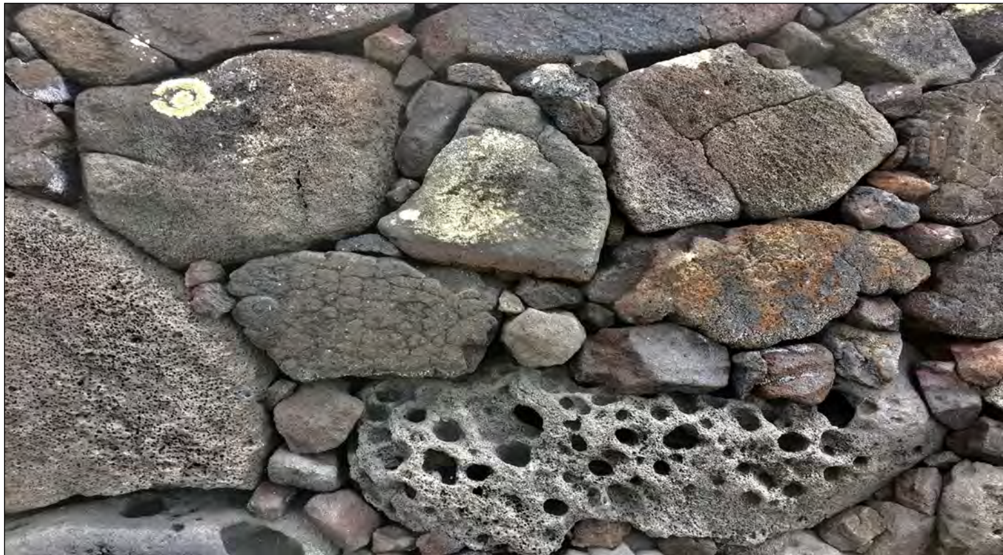
Photo: The intricate structure of a wall constructed using uhaul humu pōhaku (Hawaiian dry-stacked masonry). Source: National Park Service Photo. https://www.nps.gov/puho/learn/historyculture/preservation.htm
