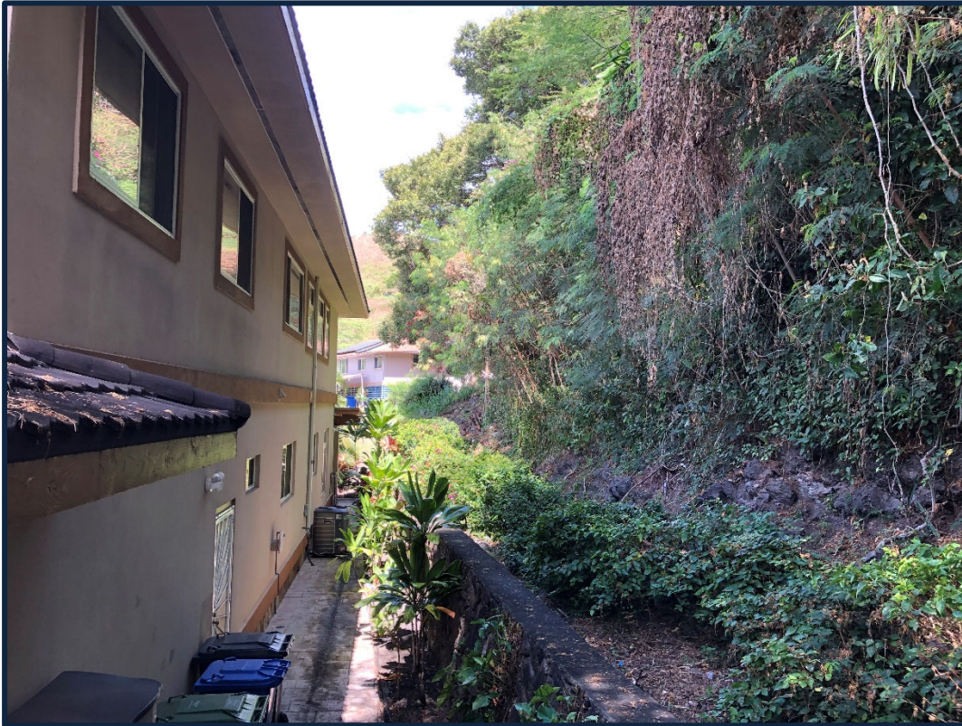
Photo No. 2 (TMK: 2-4-42: 12) – Profile view of existing CRM retaining wall. Front of wall measures approximately 5 to 5.5 feet above the top of the adjacent concrete slab. Back of wall measures approximately 1-foot above the top of the backfill.
