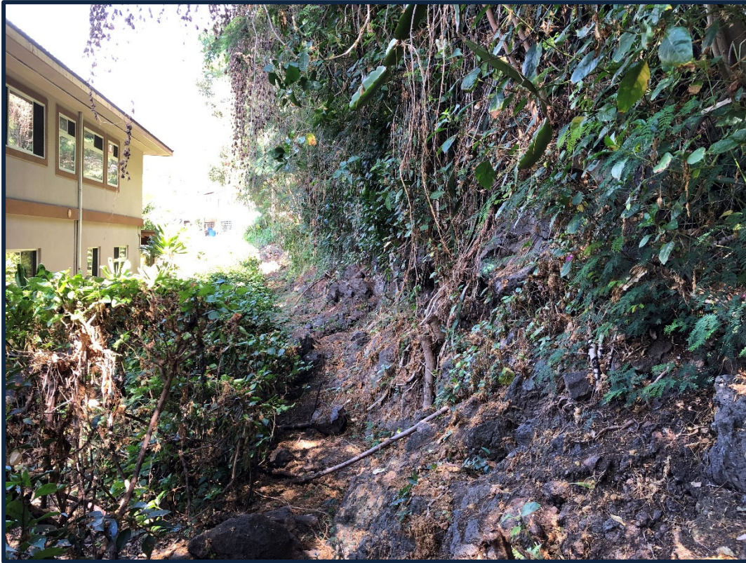
Photo No. 3 (TMK: 2-4-42: 12) – Profile view of existing slope. Rocky material exposed below heavy vegetation.
