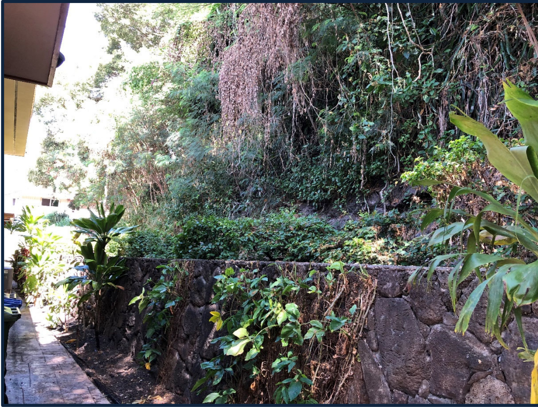
Photo No. 1 (TMK: 2-4-42: 12) – Existing CRM wall at the back of the property. Adjacent slope is highly vegetated.
