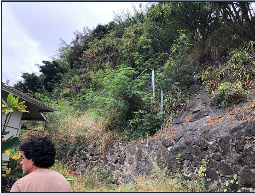
Photo No. 15 (TMK: 2-4-42: 17) – Damaged edge of fence on eastern side of the property. The approximately 2.5 to 3-foot diameter boulder damaged the fence post and top cross-brace, but the fence remained relatively intact and retained the boulder.
