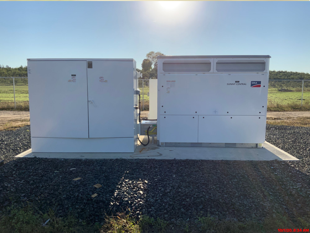
Monitoring System & Inverter
