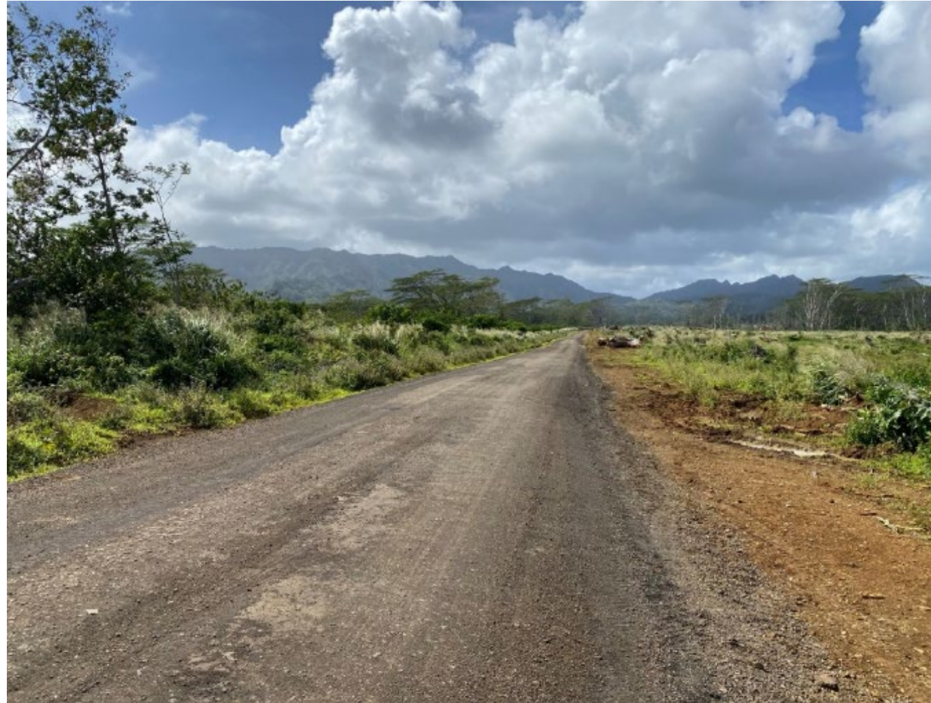
Improved roadway near southern boundary of DHHL property facing west (mauka)
