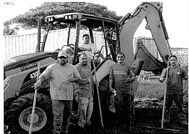
Native owned Civil Engineering firm EM Rivera & Sons' crew pictured above helping La'i'opua 2020 to install its sewer system for Phase one of the community center development plan.
