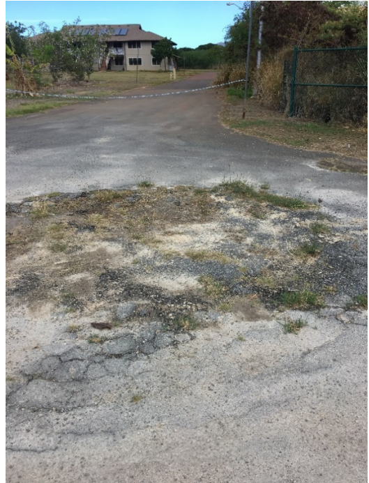
Photo 2.7. Ponding on Driveway
