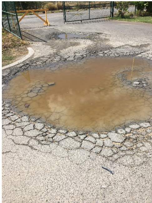
Photo 2.8. Potholes and Cracking on Parking Lot
