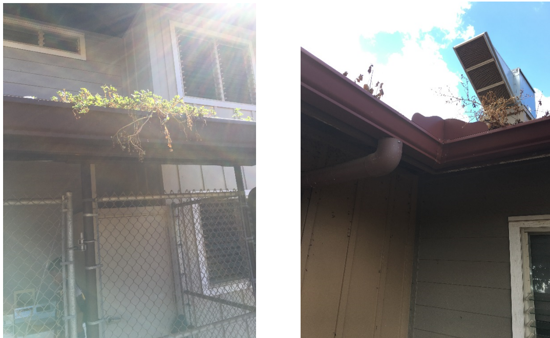
Photo 2.5. Debris in Gutters
