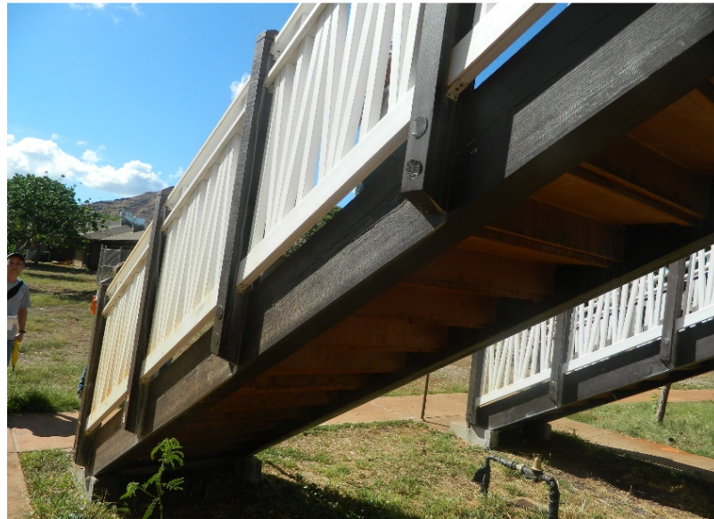
Photo 3.3. Wood Railings Bolted Outside
