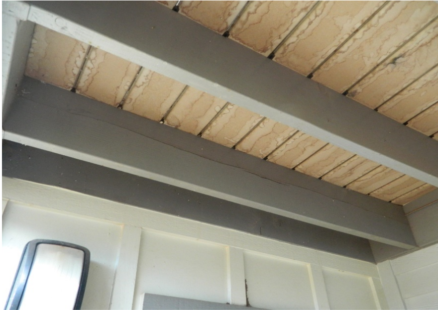
Photo 3.6. Exterior Deck Framing Joist from B205
