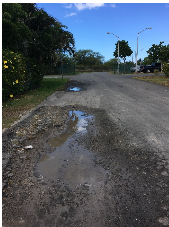
Photo 2.6. Rutting and Cracking
