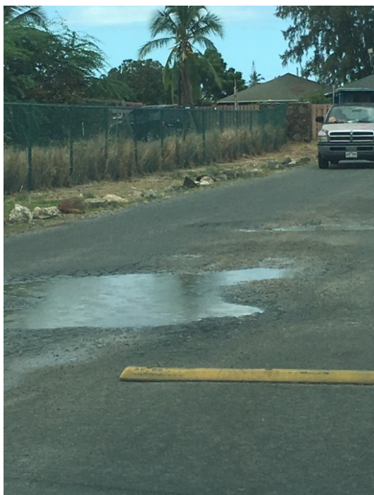
Photo 2.1. Holt Road, Asphalt Concrete Depression
