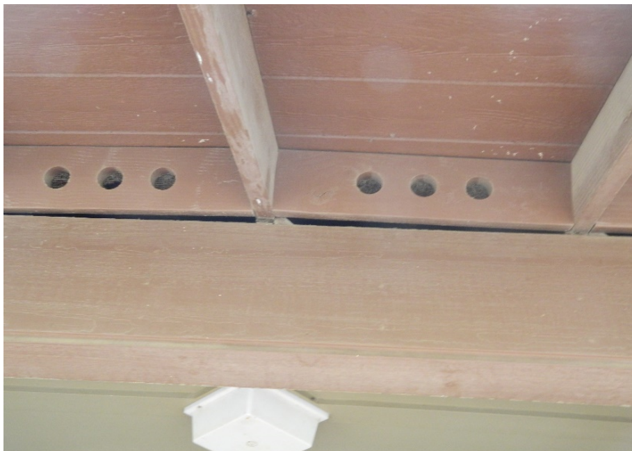
Photo 3.12. Roof Beam Gap
