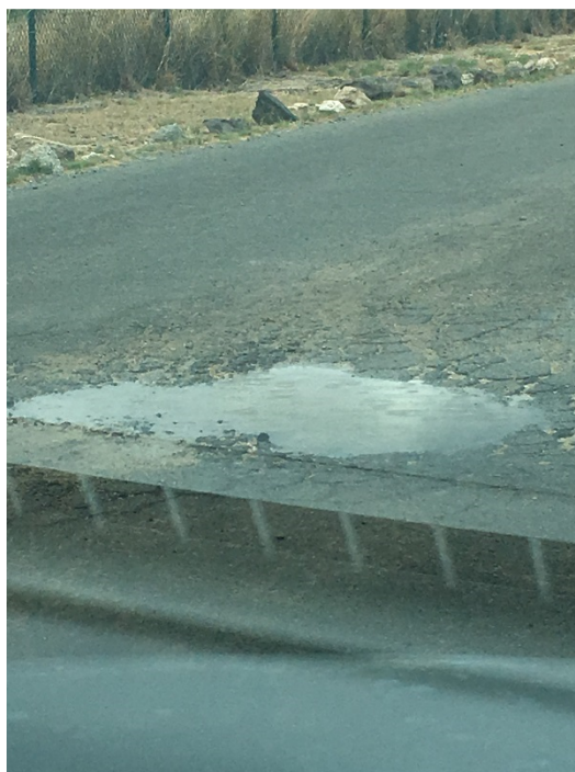
Photo 2.1. Holt Road, Asphalt Concrete Depression
