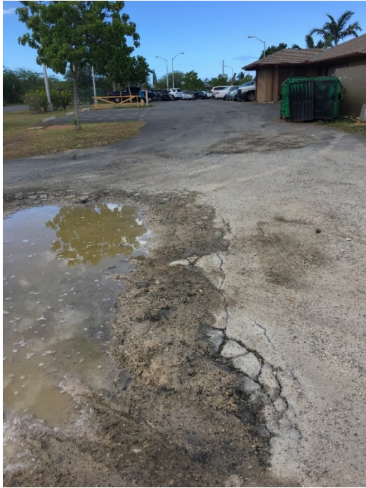
Photo 2.7. Ponding on Driveway
