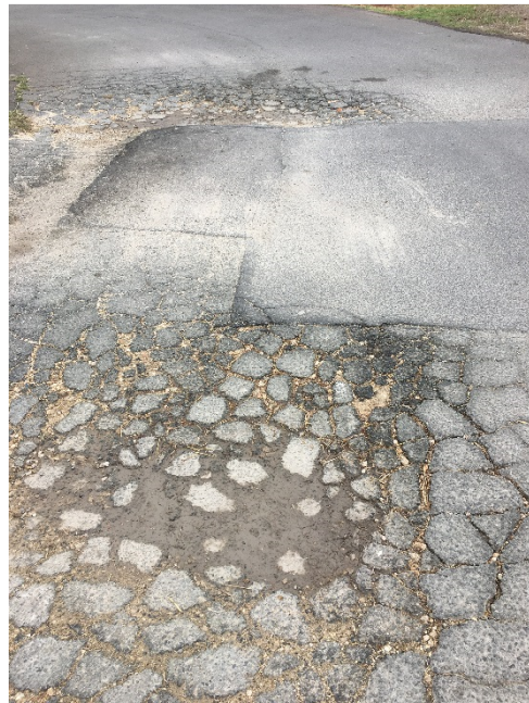
Photo 2.8. Potholes and Cracking on Parking Lot
