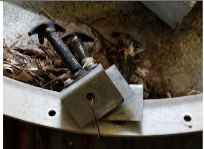
Tank Roof Cap Clamp
