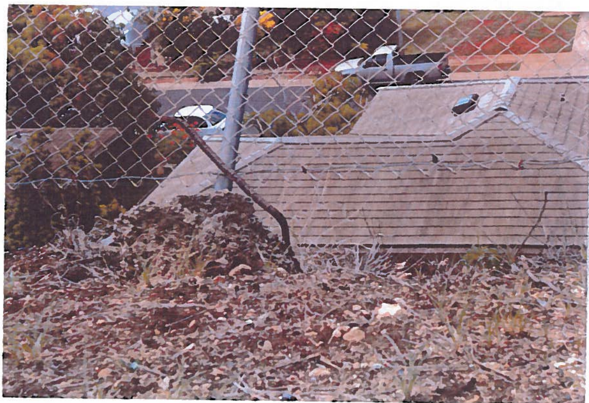
FENCE POLE HAS LOST ITS FOOTING
