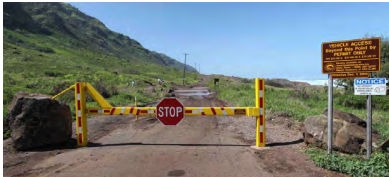
Heavy-duty security barrier gate at Ka'ena Point State Park Reserve.
