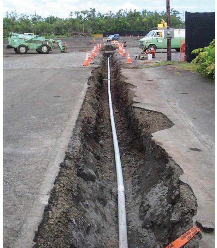
Fiber optic cable being laid at Unit 6 of the Pana'ewa Residence Lots.
