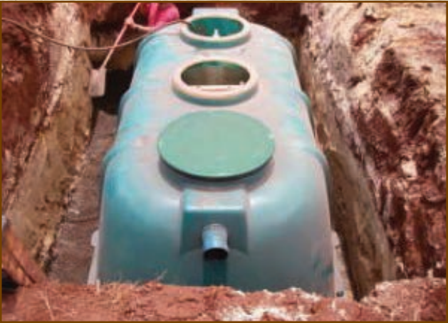
Individual Wastewater System (IWS)
