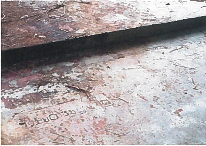
Photo 1: Identified lead hazard area from deteriorated red/gray LCP in high traffic area located on front concrete entry stairs.
