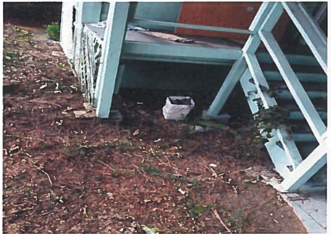
Photo 5: LCP detected on gray exterior stairs
