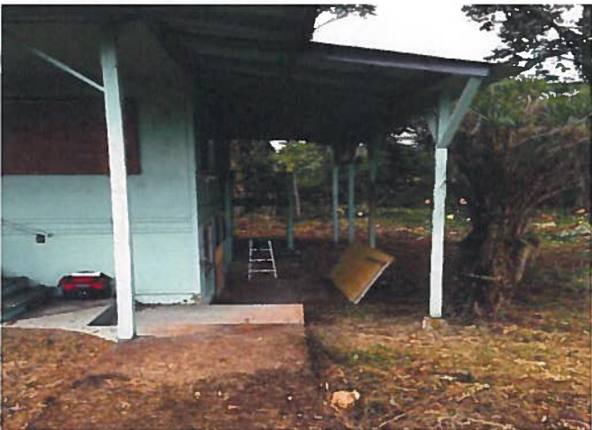
Photo 2: Exterior green wood siding and support posts in fair condition. LCP detected on gray roof fascia.
