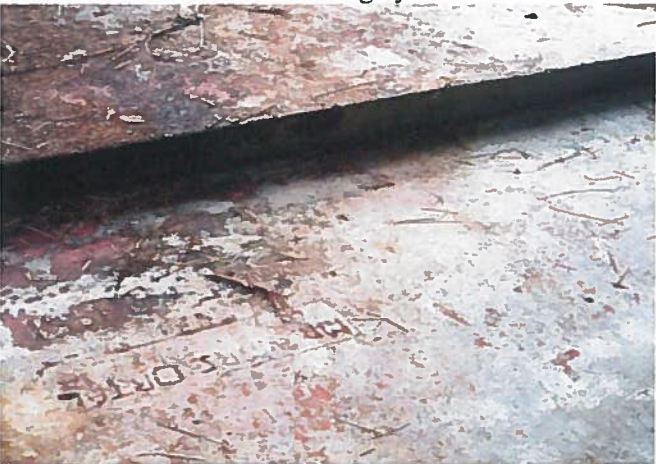
Photo 3: LCP detected in deteriorated red/gray paint located on front concrete entry stairs.
