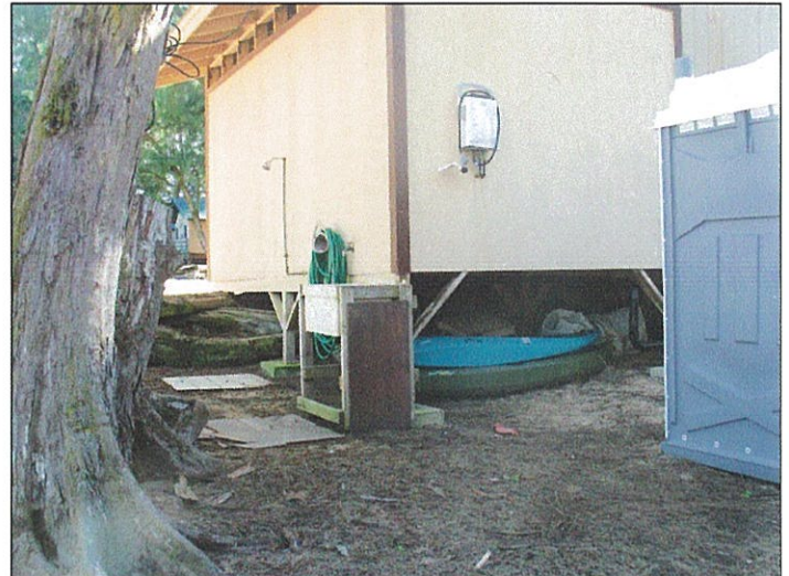
Sink and Shower Behind Restroom
