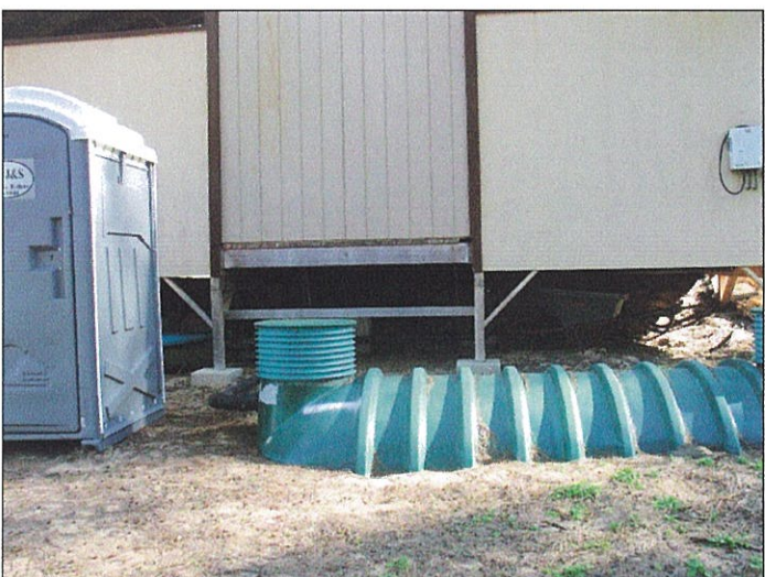
IWS at Rear of Restroom Bldg.
