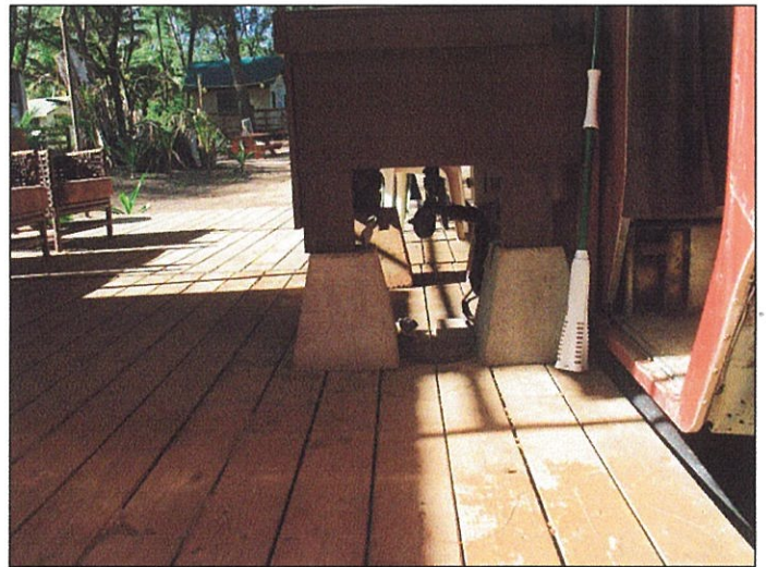
Plumbing Leading from Sink
