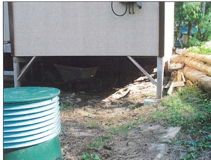
Foundation, Restroom Bldg.
