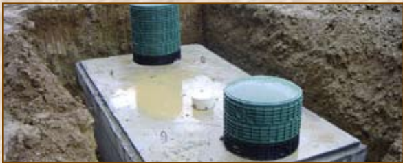
Individual wastewater system septic tank
